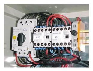
There are 1 or 2 (depending on the model) overload trip switches on the LHS of the fuse box, marked Q1 & Q2. Check the the black switch(es) are are vertical (as shown in photo above). If not, reset switch (es).
