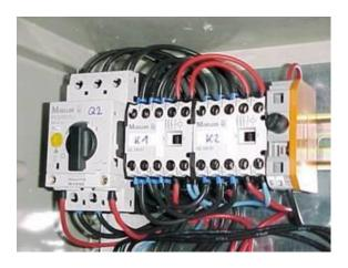
There is a fuse on the RHS – unscrew and check it is OK. If OK, put back in. Otherwise, have store electrician replace fuse. If a fuse has blown, the machine has to have drawn extra power for a reason – load unbalanced, trolley or rolls jammed under machine, something jammed in a chain, etc. Check machine carefully to make sure there are no jams anywhere before operating it again.
